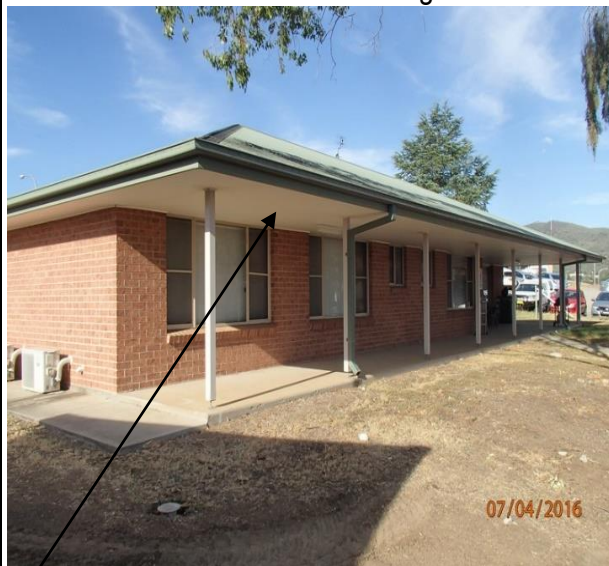
PHOTO N°2: Verandah Soffit Lining
