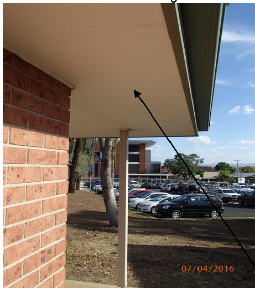
PHOTO N°1: Eave Soffit Lining
